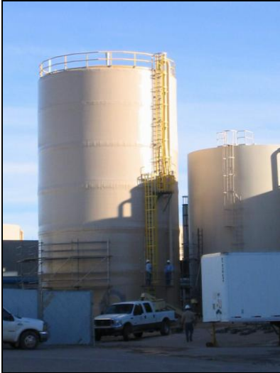
Completed 350,000 gallon tank
