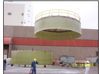
Setting top section with handrail
