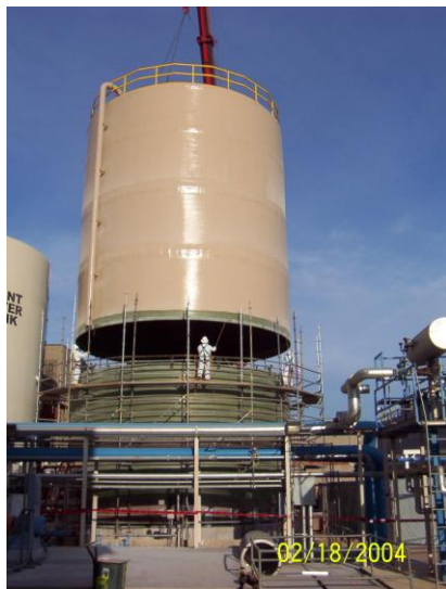
Setting upper sections on lower sections
