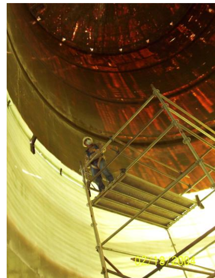
Interior seams applied & inspected
