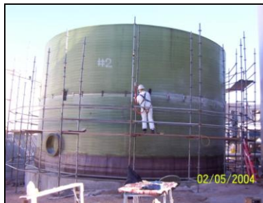
Assembly of lower sections
