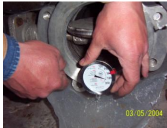
Checking temperature during steam cure
